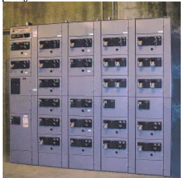
In addition to motor control panels, motor control centers can be furnished as part of the control package.
